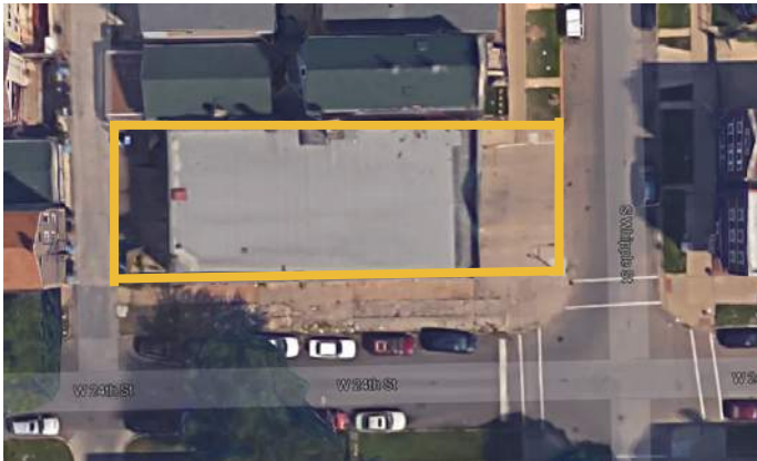
▲ Site aerial view (above)
